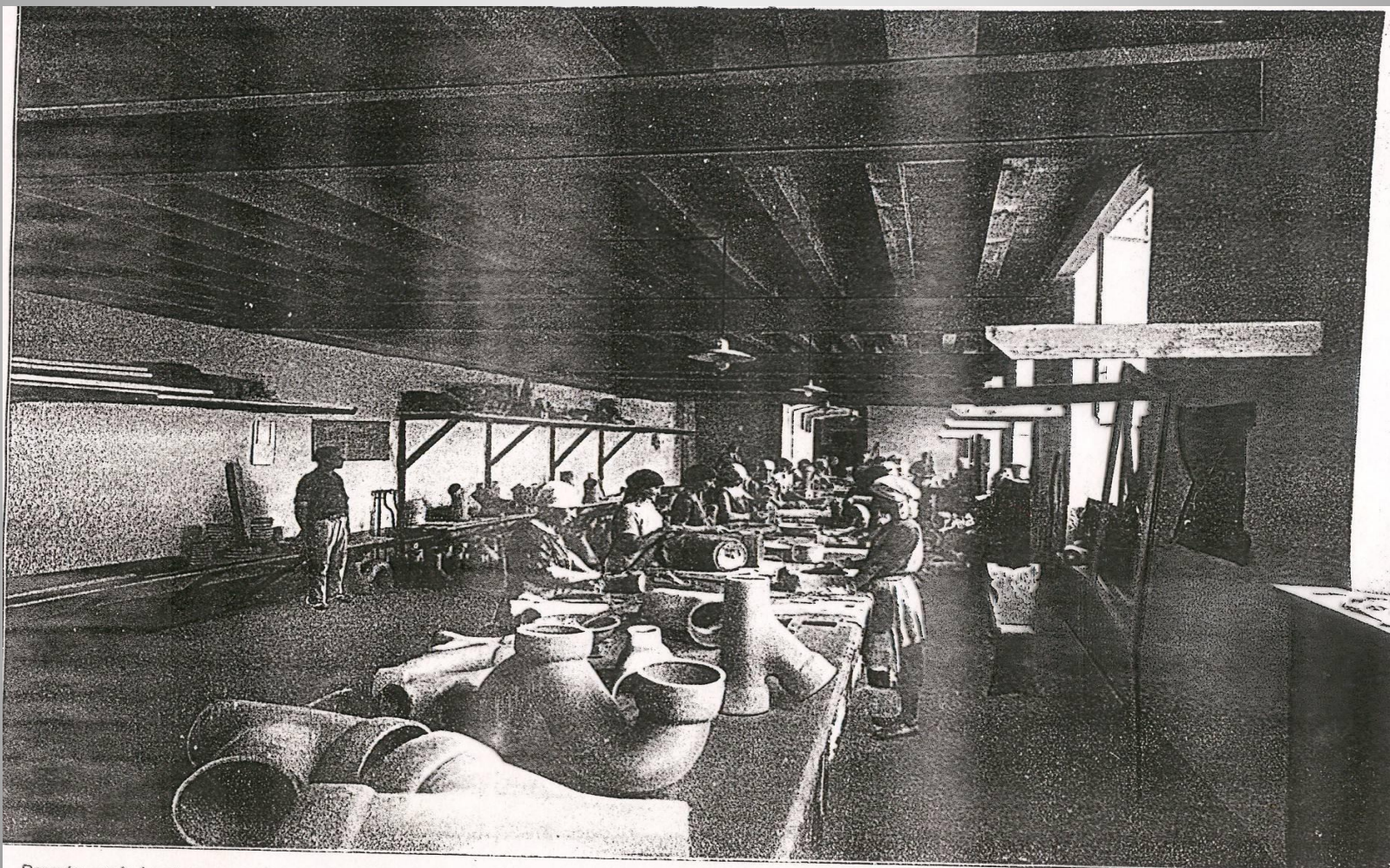
Section for making Eternit fittings, for drainage conducts.
