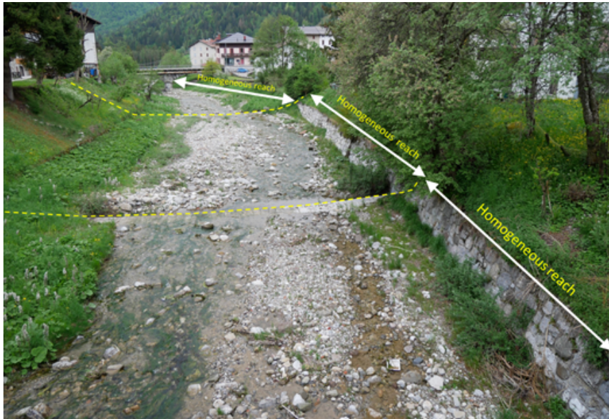
Figure 35. Example of mountain river subdivided in homogeneous reaches. In this case, the first subdivision is due to the presence of a hydraulic work, while the second is due to changes in the river flank morphology.
